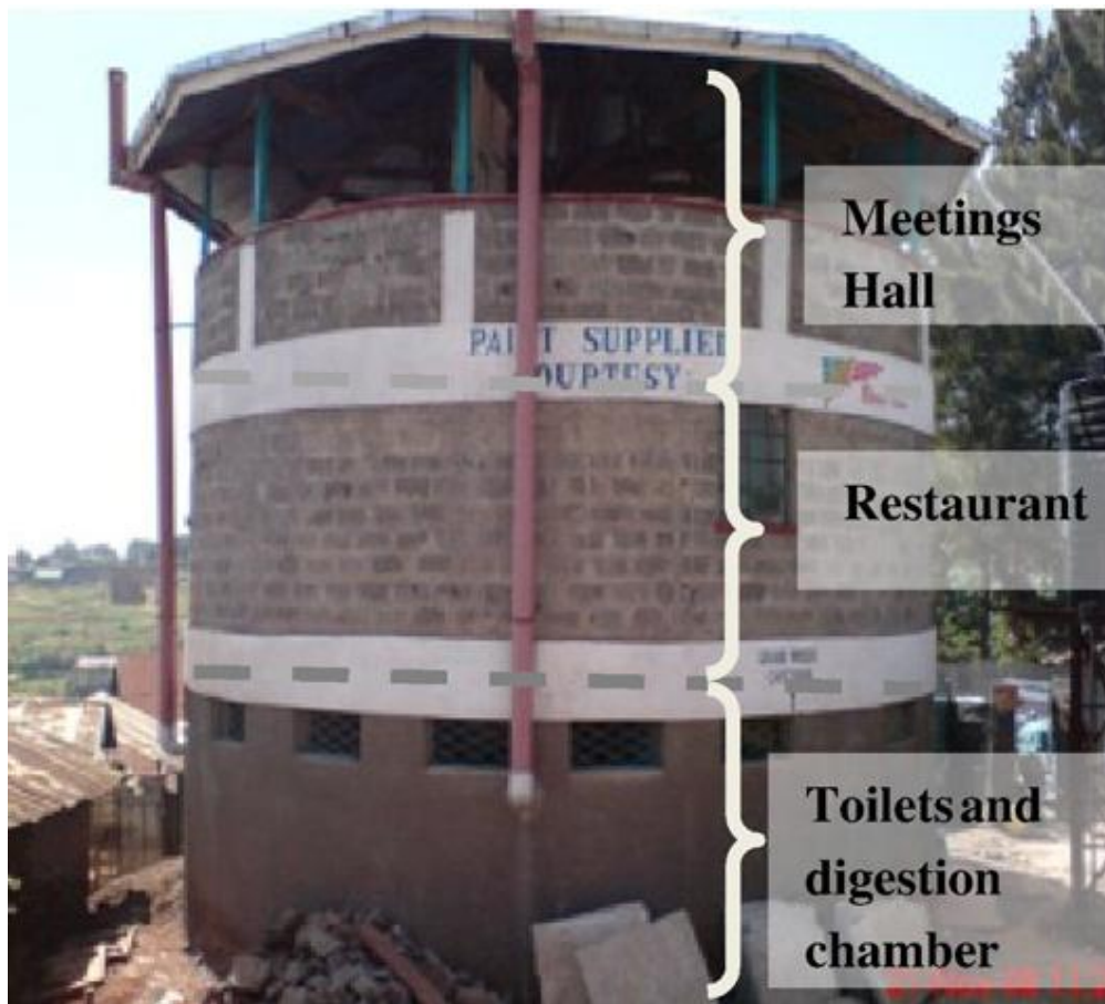
Fig 4 Bio gas toilet system in India
